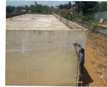
Repaired existing government run school building
